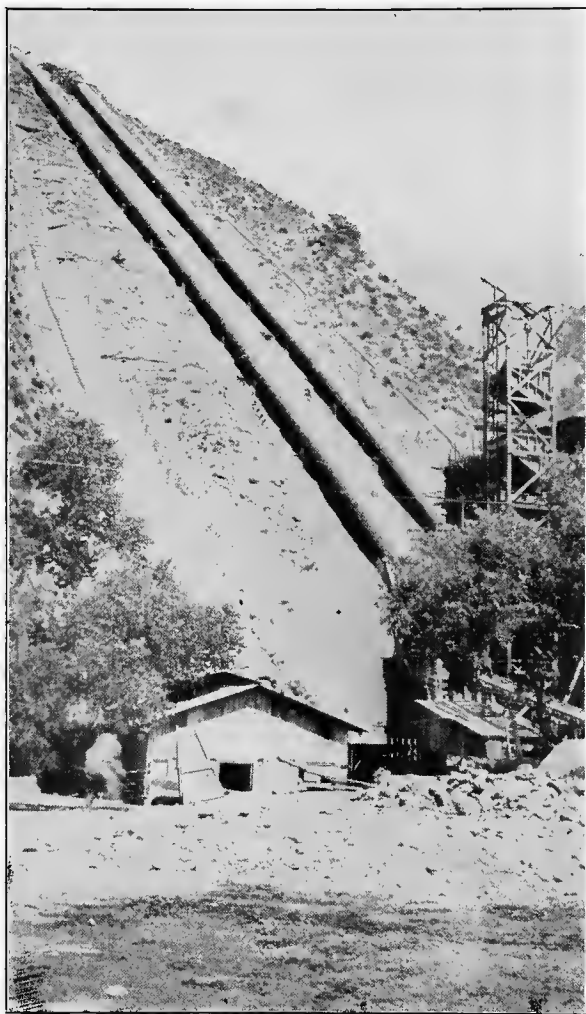
Penstocks—City of Los Angeles
